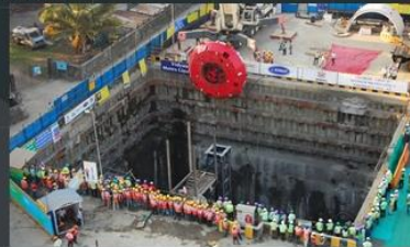
TBM being lowered
