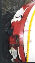
Cutting through rock
