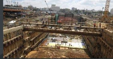
Underground Metro Station under construction
