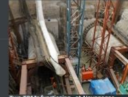
Two TBMs functioning at Nayanagar
