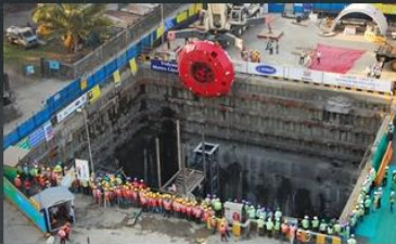
TBM being lowered
