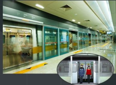
Example of an underground Metro Station with safety doors
