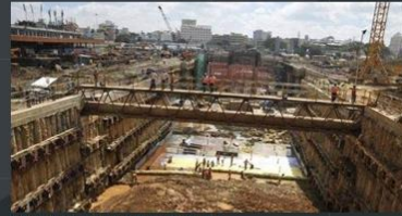
Underground Metro Station under construction
