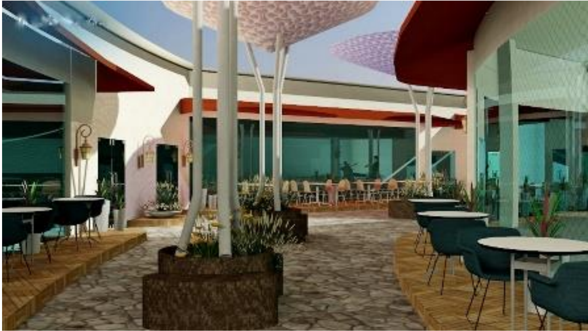
Mall Terrace Architecture
